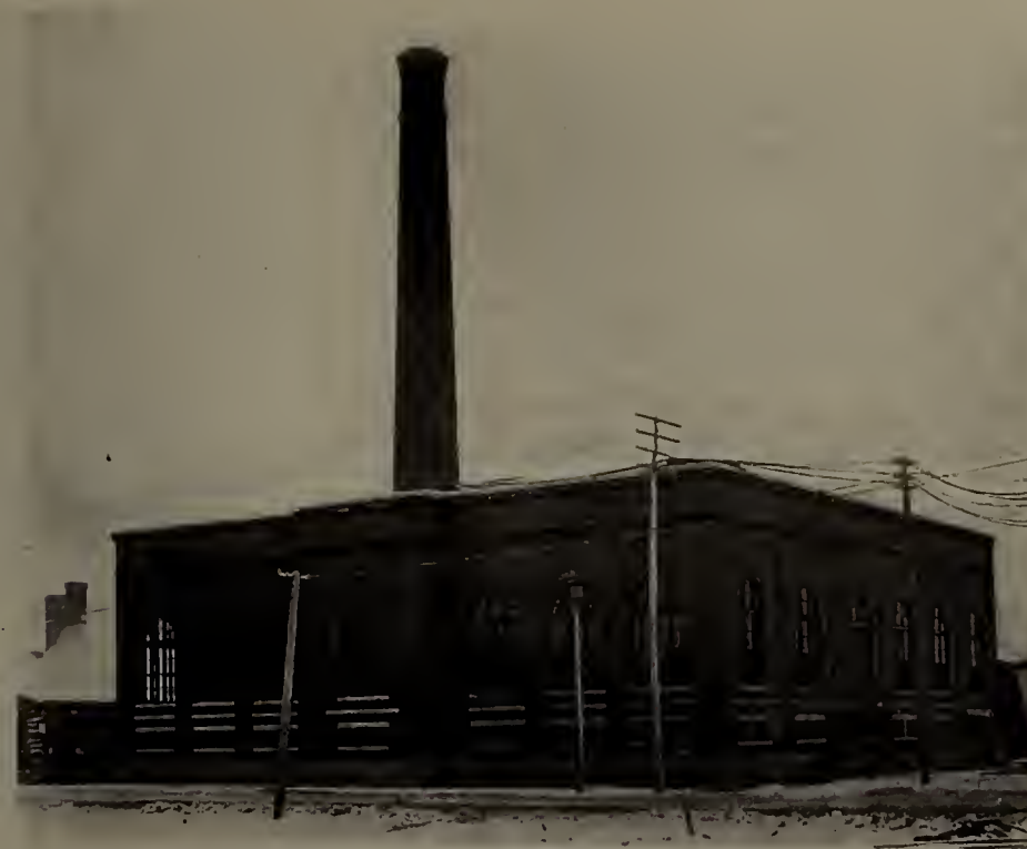
POWER PLANT FOR THE PORTLAND RAILROAD COMPANY, Portland, Me. Designed by Sheaff & Jaastad, Engineers, 85 Water Street, Boston.
